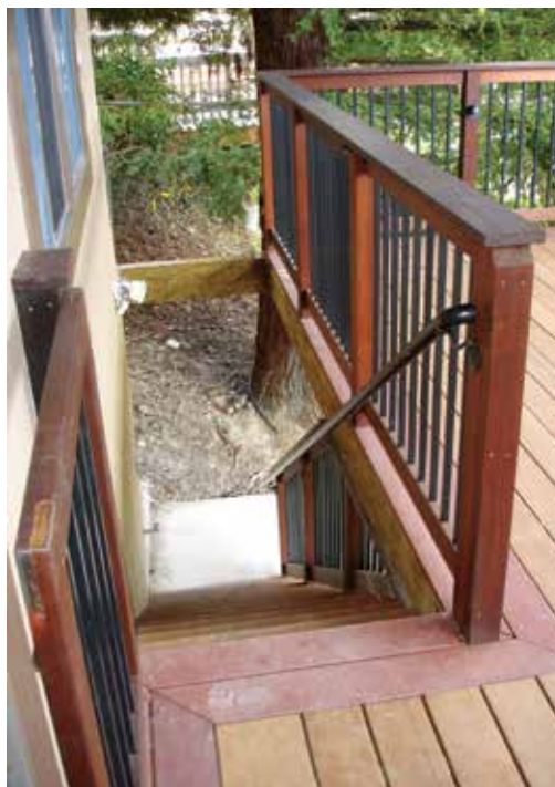
Figure 8. The deck's posts and rails were made from ipe and fitted with square aluminum balusters.
