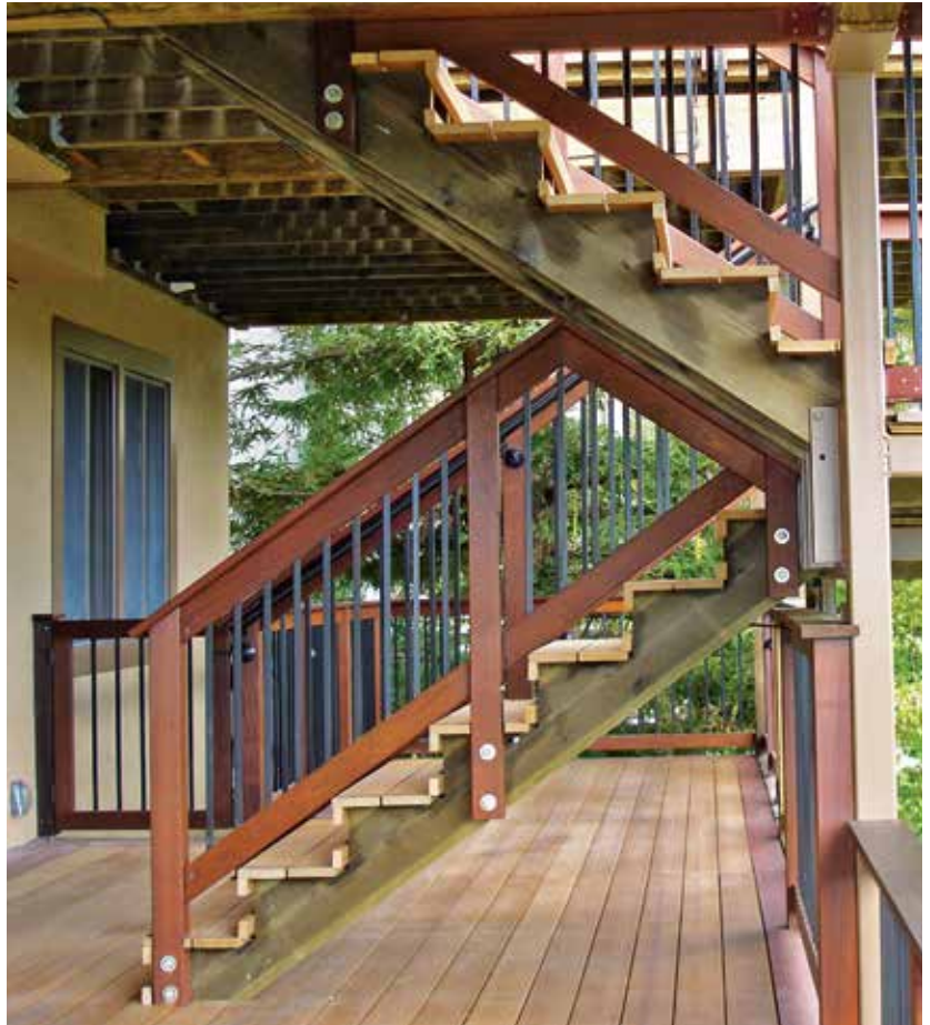
Figure 8. The deck's posts and rails were made from ipe and fitted with square aluminum balusters.
