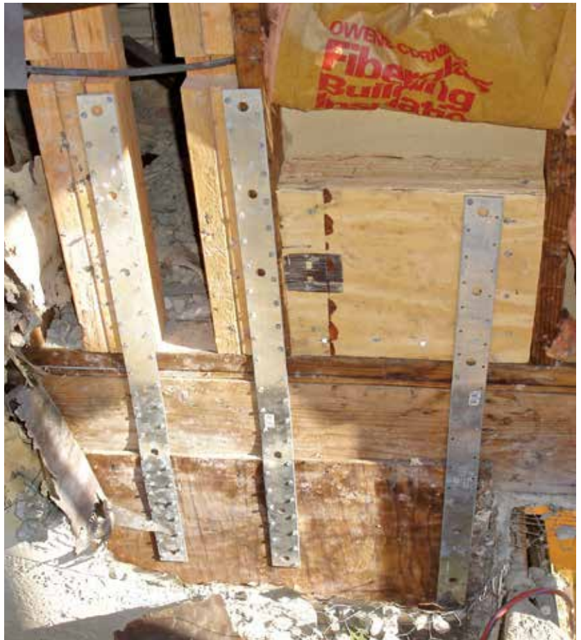
Figure 4. Multiple DTT2 tension ties were specified by the engineer for the ledgers at each deck level to help resist lateral loads.
