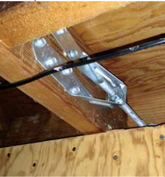
Figure 4. Multiple DTT2 tension ties were specified by the engineer for the ledgers at each deck level to help resist lateral loads.
